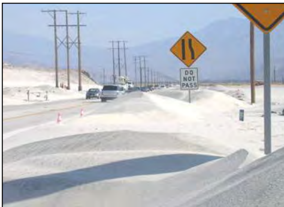
Windblown sand hazard along Indian Canyon Drive.
